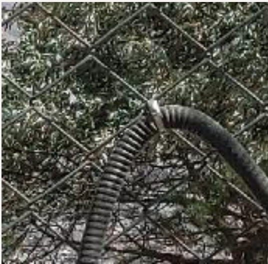
Armored microphonic cable with cable tie for connecting the cable to fence
