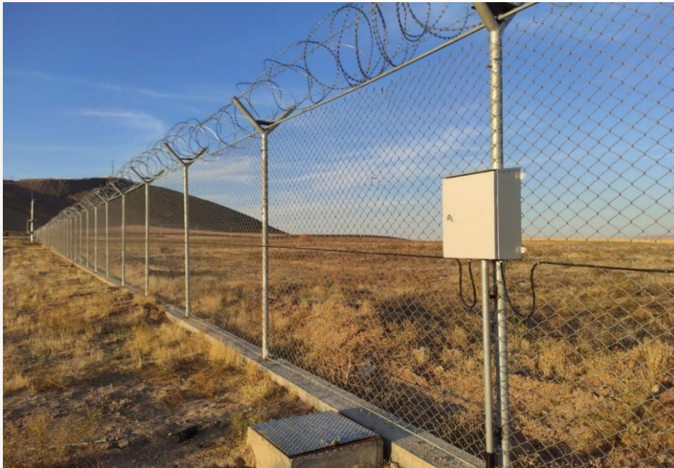
Installed Microphonic cable on a conventional fence
