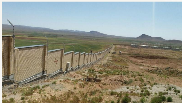
Installed Smart electric fence
