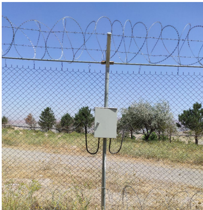
Microphonic sensor cable and Analyzer installed on a conventional fence
